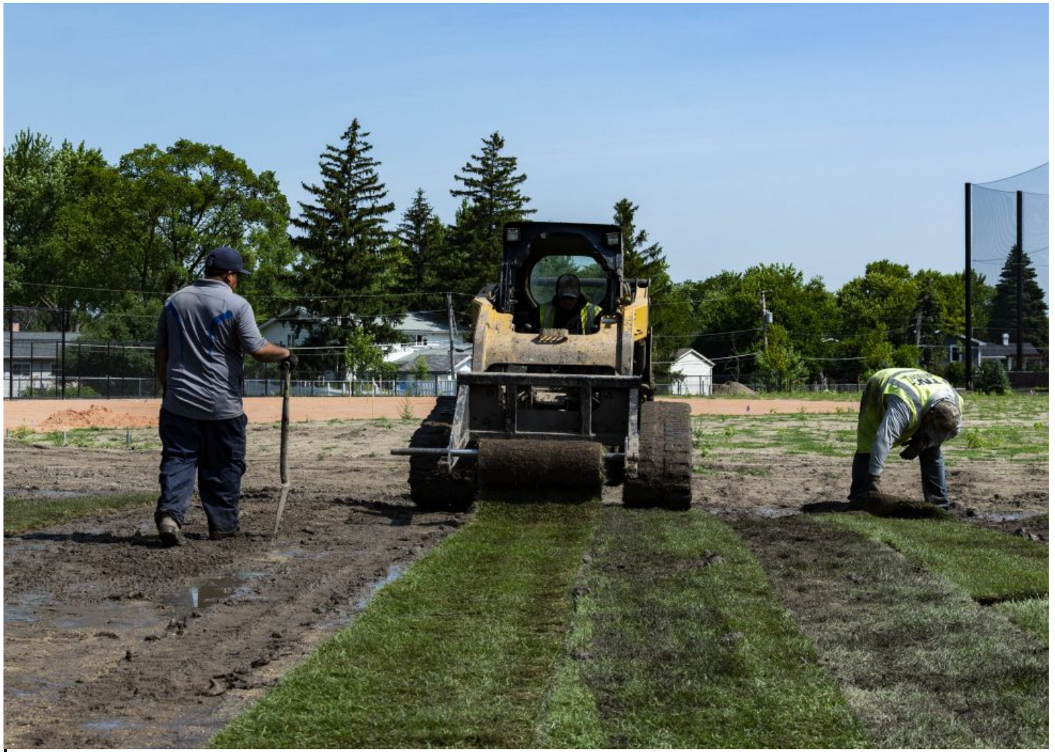
Crews lay sod in the outfield of James B. Conant High School's baseball outfield.
