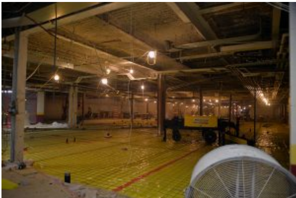
The floor is prepared for concrete.
