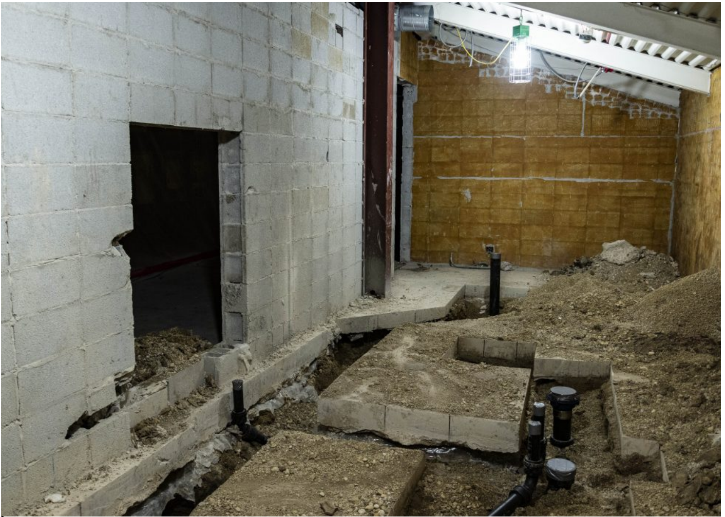
A bathroom at James B. Conant High School which has been torn down in preparation for a complete overhaul.
