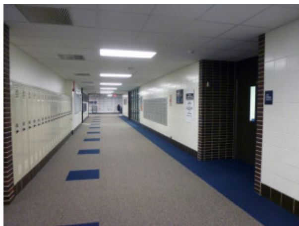
Lockers will be removed from where the main offices are located to increase student safety and update original building construction from 1962.
