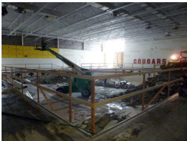
CHS' pool renovation
