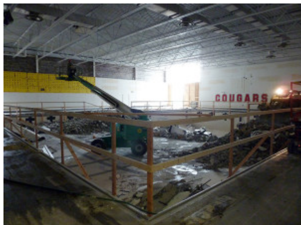
CHS' pool renovation
