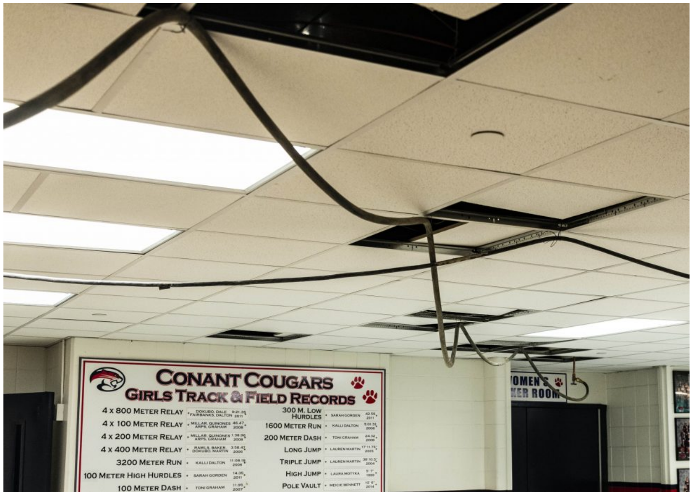
Temporary water lines span the ceilings of James B. Conant High School during construction on the school's bathrooms.
