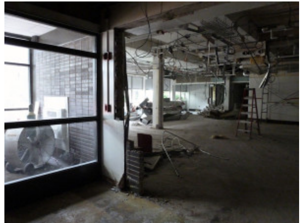
CHS' front entrance and main office are under construction
