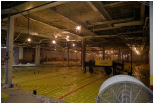
The floor is prepared for concrete.
