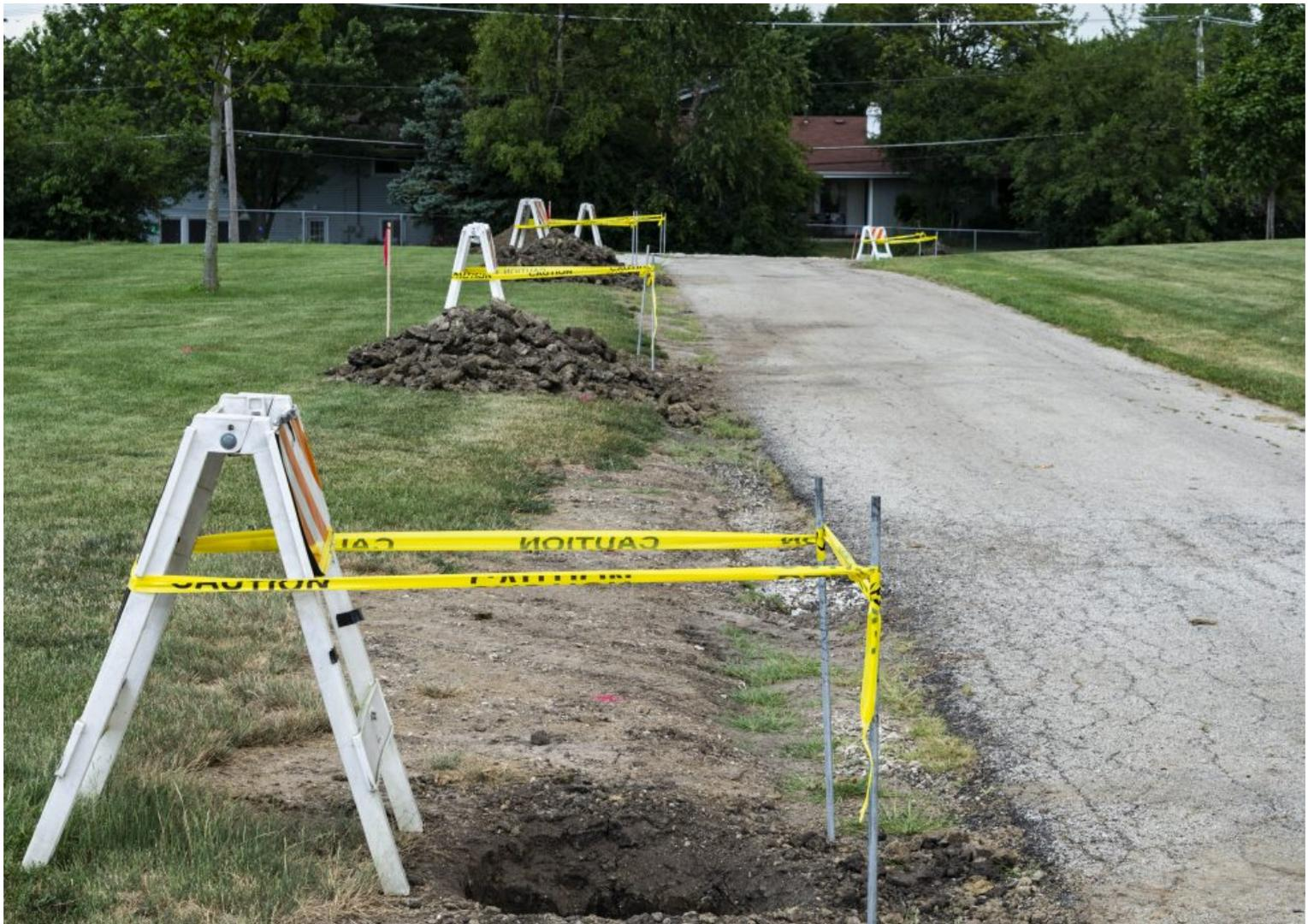
*Crews dug out post holes for the installation of new safety lights between the fields at Hoffman Estates High School.*
